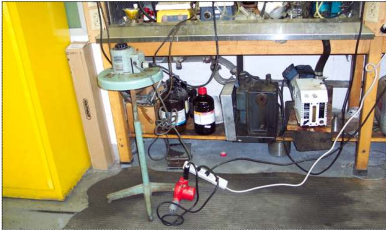
Fig 5.1.3 Liquid spilled on carpet floor with tools and equipment around
